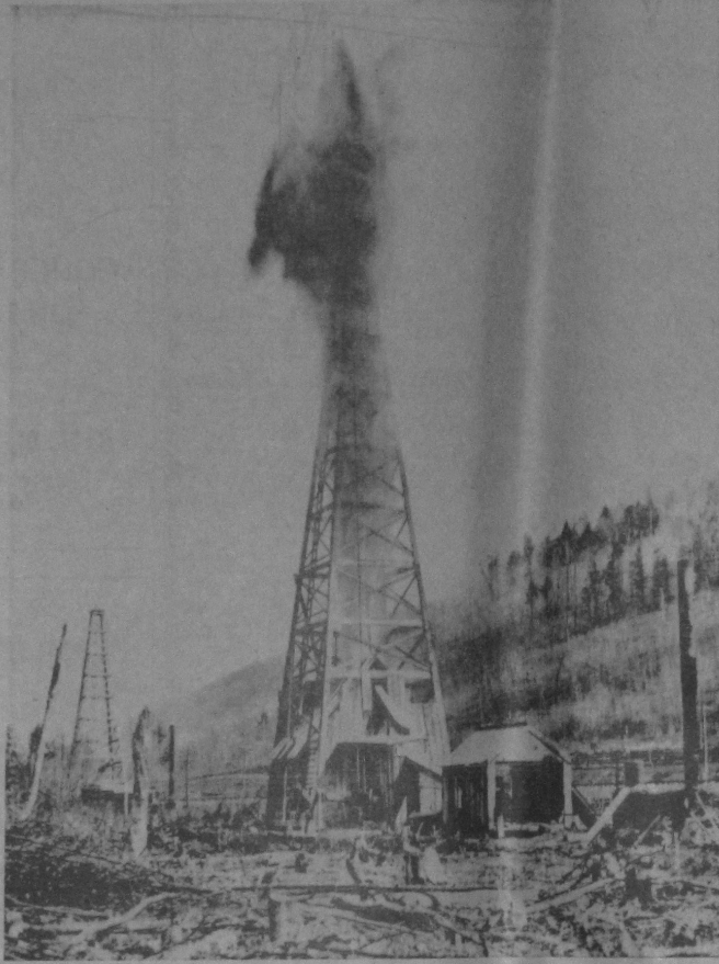
SHOOTING AN OIL WELL in the 1890s — familiar sight on the Bradford Field horizon over the years. Note a second derrick in left background and the boiler in right foreground.
